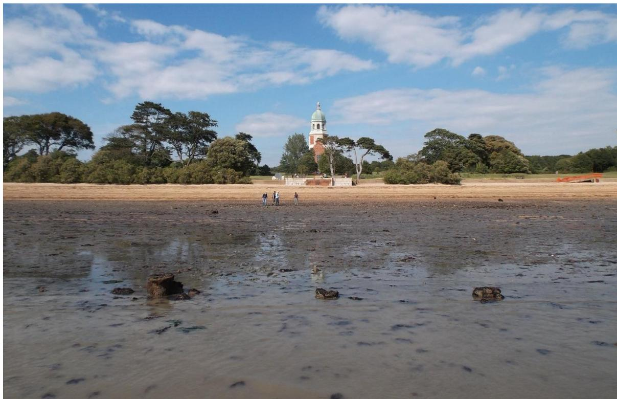
Figure 8. View from the water's edge north-east towards the pier entrance along the central axis of the pier. A complete bent of pilings is visible in the foreground with a spacing of eight foot between piles.
