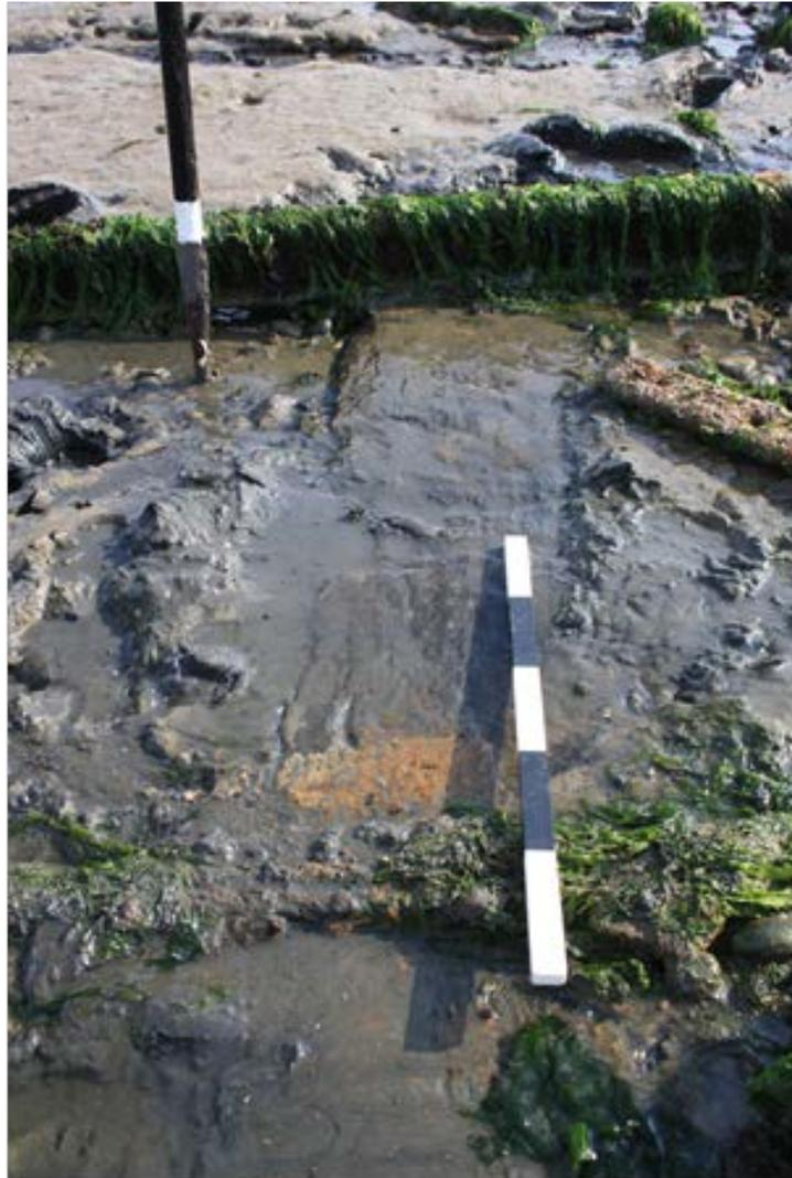
FIGURE 55: ONE OF THE SLEEPERS WHICH PROVIDE THE FOUNDATIONS FOR THE RAILS OF THE NORTHERN SLIPWAY
