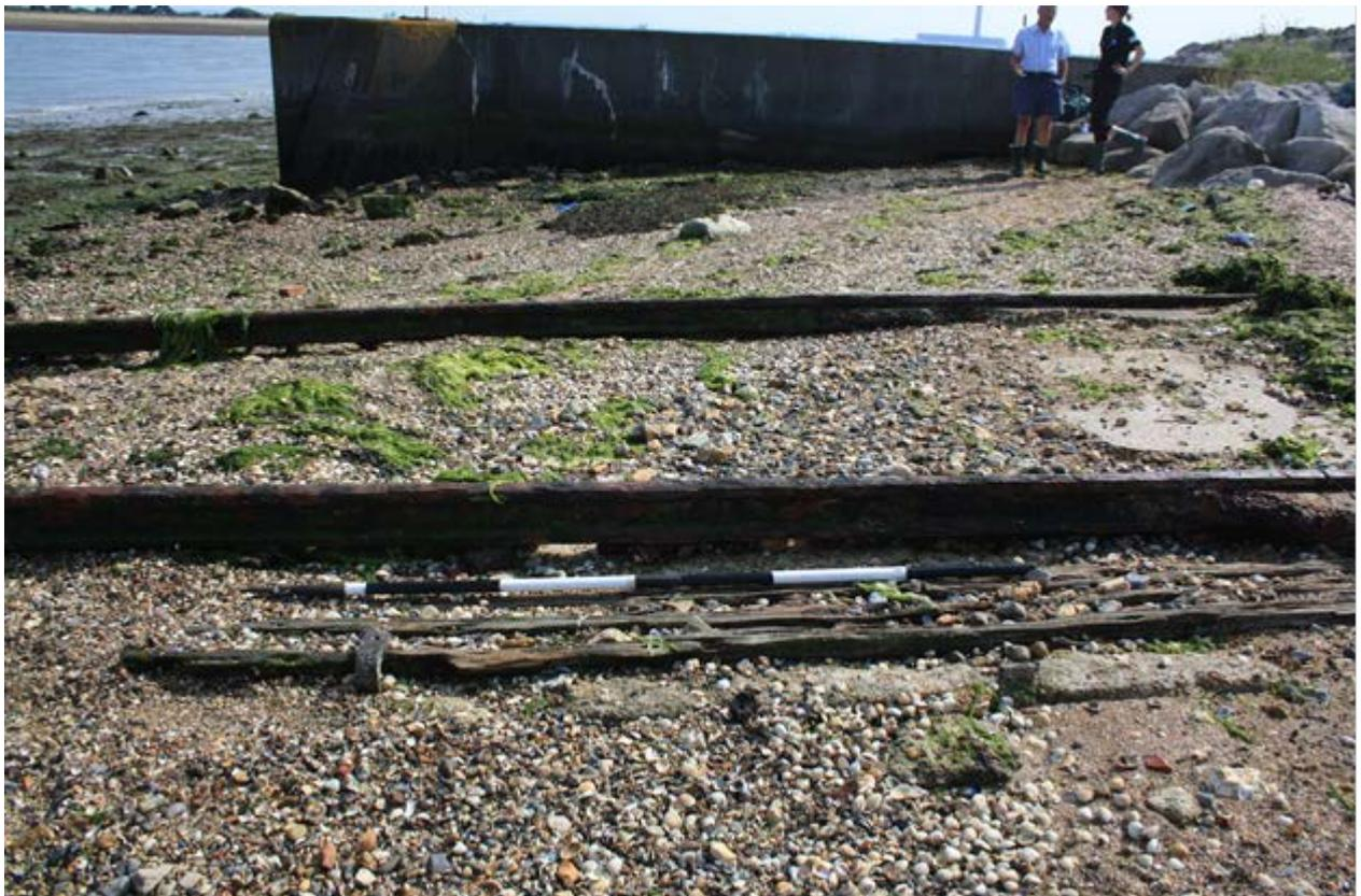
*FIGURE 57: THE CONCRETE AND WOODEN FOUNDATIONS OF THE SOUTHERN SLIPWAY RAILS*
