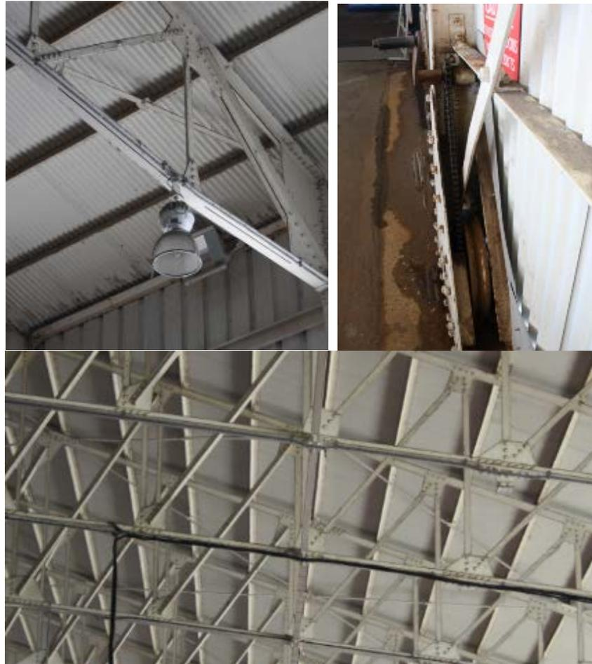
FIGURE 19: INTERNAL FEATURES OF THE SUNDERLAND HANGAR. TOP LEFT: LIGHTS. TOP RIGHT: SLIDING DOOR MECHANISM. BOTTOM: STEEL CEILING.
