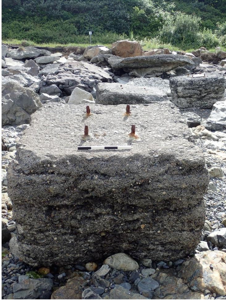
*FIGURE 85: CONCRETE SECTION WITH IRON FASTENINGS WHICH COULD HAVE FIXED A HANGAR STANTION*
