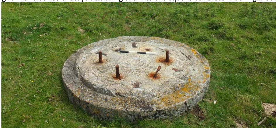
FIGURE 4.23: CIRCULAR FOOTING OF MAST
