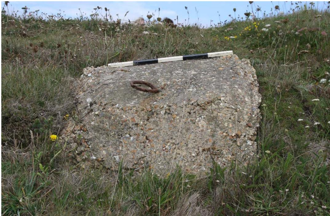
*FIGURE 4.59: CONCRETE BLOCKS WITH MOORING RINGS FOR THE WIRELESS MAST STAYS*
