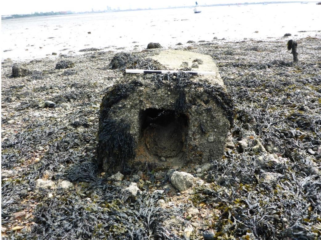
FIGURE 4.48: CROSS SECTION OF ONE OF THE PIER LEGS WITH WOODEN REMAINS IN THE CENTRE. 50CM SCALE.
