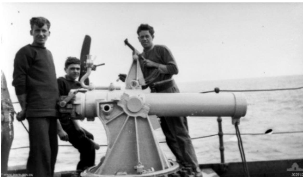
Figure 11: 7.5 inch naval howitzer on board *SS Orca*
